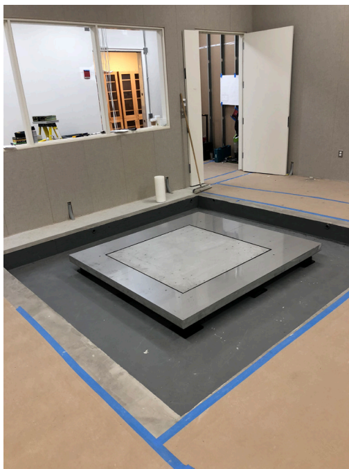
The images above represent a successful recessed floor platform for a TEM vibration isolation platform, TEM acoustic enclosure, and TEM HT Tank vibration isolation platform.
