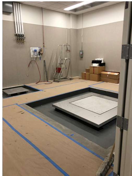
The images above represent a successful recessed floor platform for a TEM vibration isolation platform, TEM acoustic enclosure, and TEM HT Tank vibration isolation platform.
