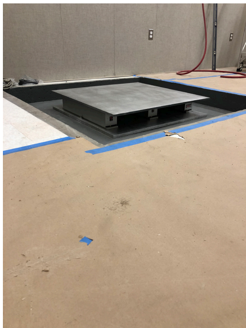
The images above represent a successful recessed floor platform for a TEM vibration isolation platform, TEM acoustic enclosure, and TEM HT Tank vibration isolation platform.
