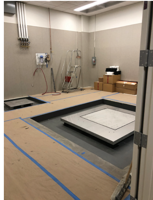
The images above represent a successful recessed floor platform for a TEM vibration isolation platform, TEM acoustic enclosure, and TEM HT Tank vibration isolation platform.
